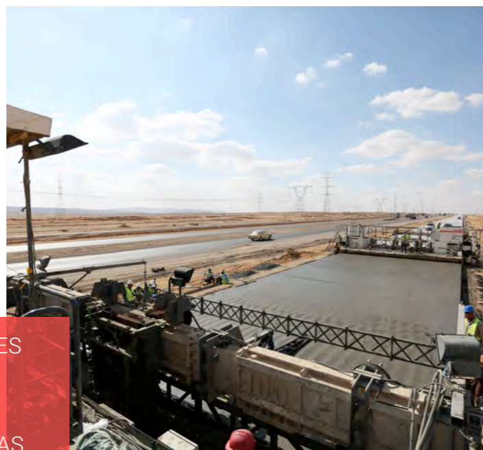
EGYPT'S FIRST CONCRETE HIGHWAY
