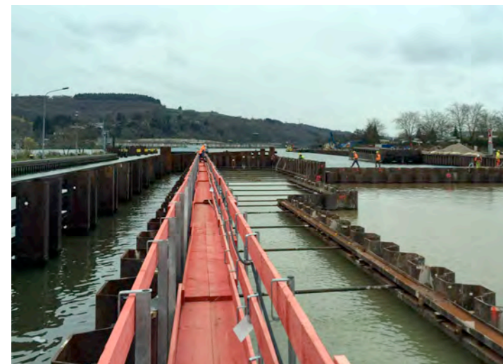
SECOND LOCK CHAMBER OF THE MOSELLE RIVER IN TRIER, GERMANY
