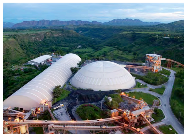
IBAGUE CEMENT PLANT IN COLOMBIA
