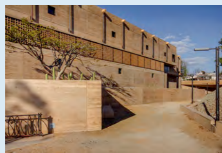
Special Prize: Construction Innovation Oaxaca's Historical Archive Building. Santa Lucía del Camino, Mexico
