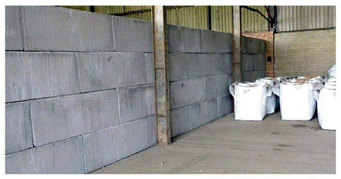
The council needed to create two additional storage bays, each to be used to segregate recycling before it is processed. The bays, measuring 16m deep by 3m wide, required one hundred and seventy of Elite Precast Concrete's Vee™ interlocking blocks to complete the project. The blocks were linked together along the base, sides, and top and formed a highly stable structure.
