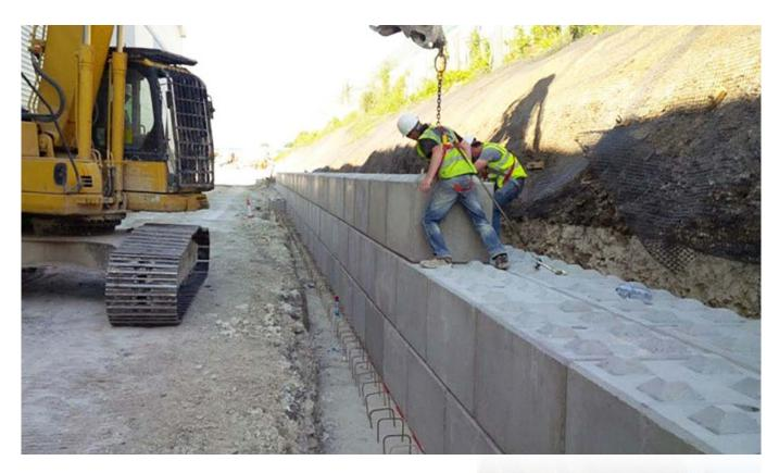
The project required a 220m long by 5m high retaining wall to be built, with Gabion baskets originally specified to create the wall. However, after careful consideration the Elite Legato® interlocking block system was chosen as this provided a quicker, space saving and overall better value solution. The finished wall consisted of over a thousand 2,400kg Legato® interlocking concrete blocks.
