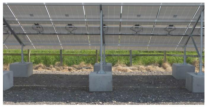
EnergyMyWay designed, supplied and installed the 152x 250-watt photovoltaic solar panels for the new building – which is set to house more than four million books, while Elite Precast Concrete's Kentledge blocks acted as counterweights and have been used to provide the system with a greater degree of stability.
