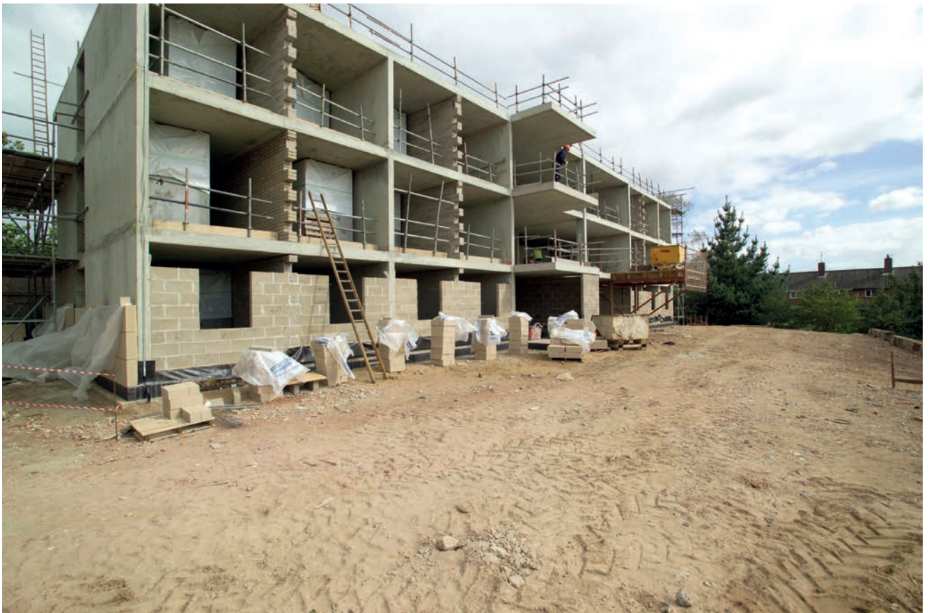
Using concrete and masonry construction limits the risk of devastating fires during construction.
