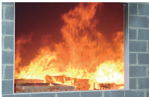
BRE used masonry walls to provide the fire containment for its full-scale hollowcore floor fire tests because of masonry's fire performance credentials.
